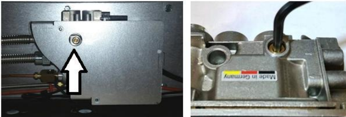
Location of Low Pressure Adjust Screw (Under the fireplace)
